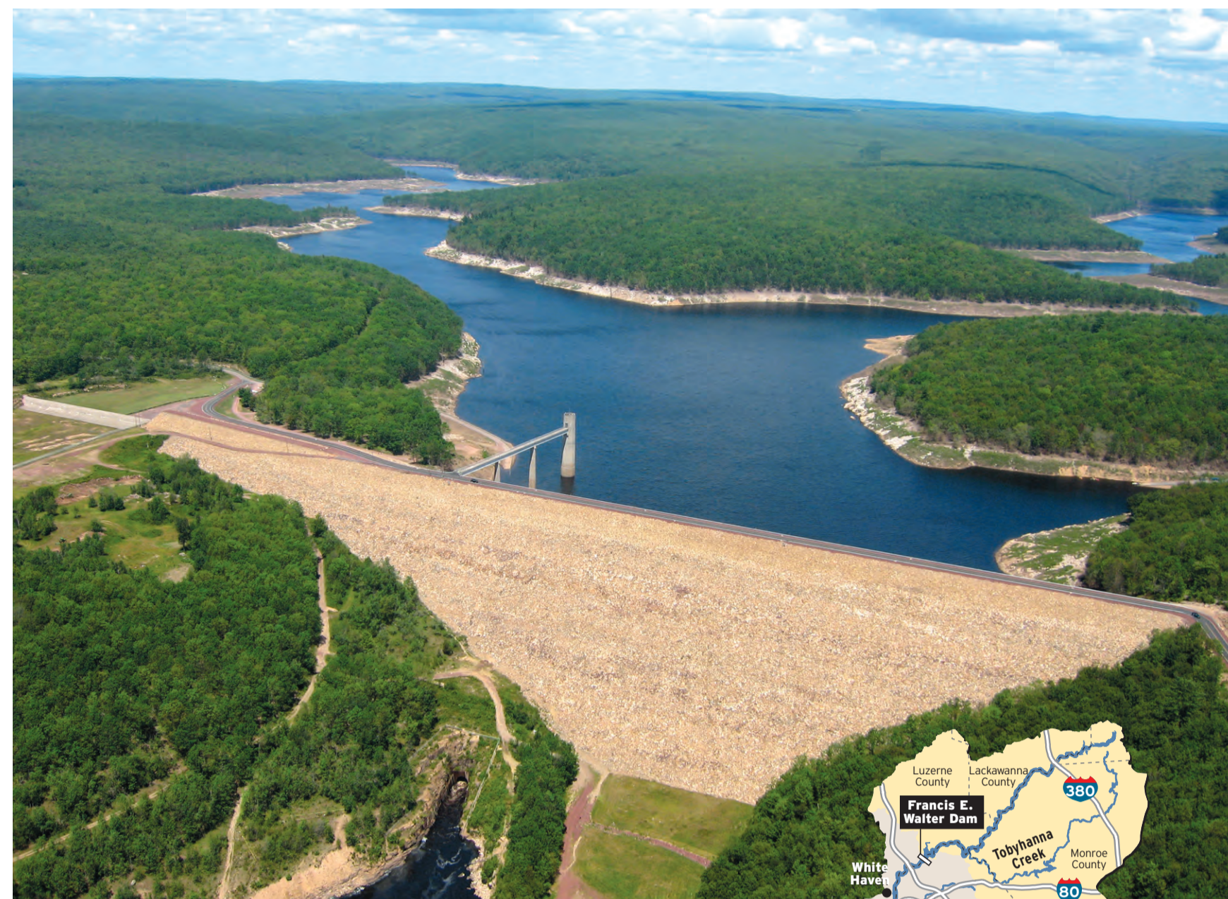
Aerial view of the Francis E. Walter Dam in lower Luzerne County (summer 2006). The release gates are located at the bottom of the release tower shown in the water (left of center).
